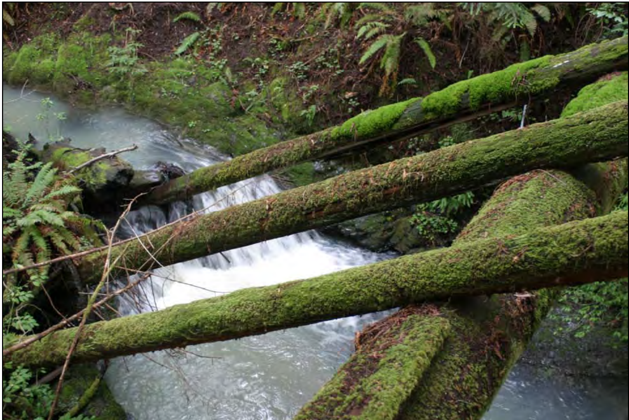
Figure 1-2. Remnant Dam Structure on Hazel Gulch
