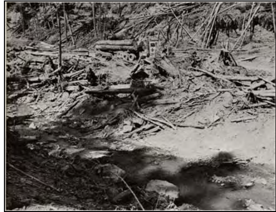
Figure 1-6. Typical 1960s Stream Crossing Through Mainstem Big Salmon Creek, Possibly Located Near Elliot Road (SFPWM 1965-66).
