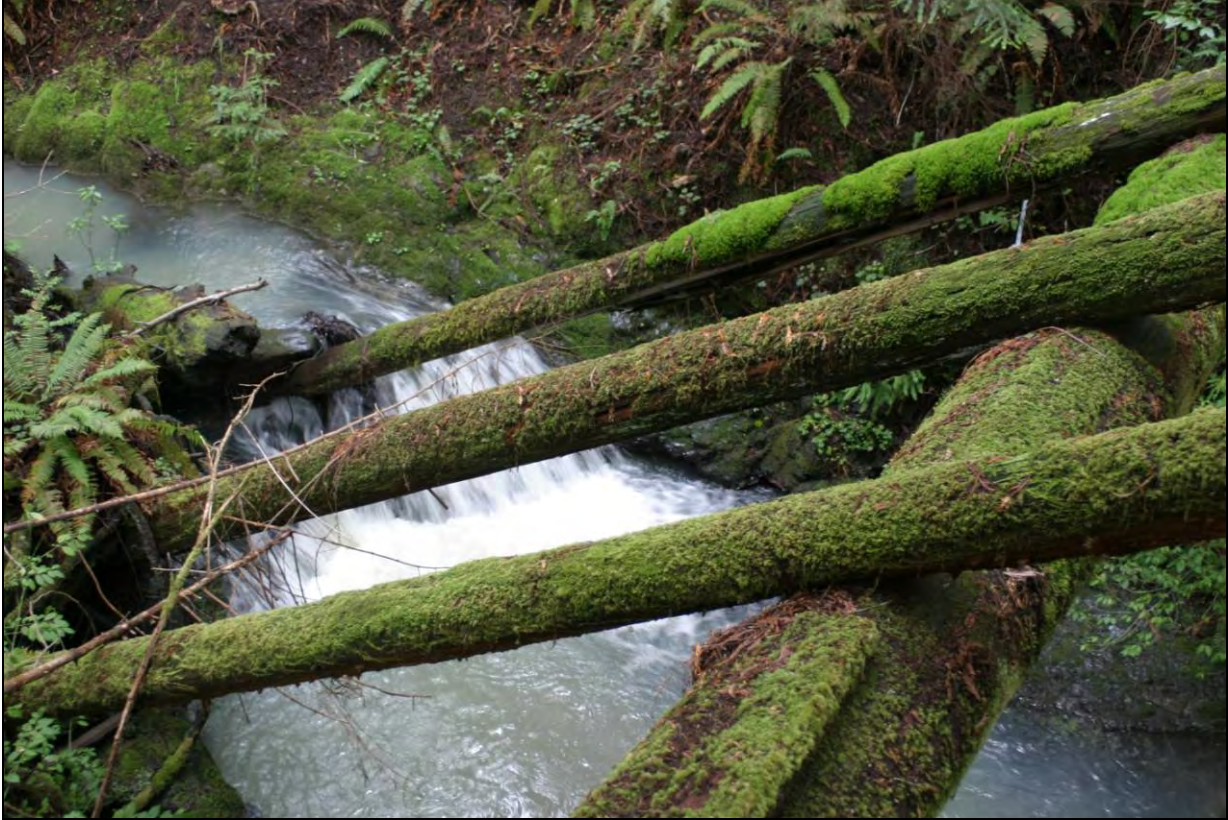
Figure 10: Remnant Dam Structure on Hazel Gulch, Circa 1998. Although dams were constructed for log and ranch ponds at various locations within the channel, splash dam logging, or stream-based log drives, did not significantly occur in the Big Salmon Creek watershed. Logs were moved to the coast mill by railway. A remnant dam structure can still be observed just above the confluence of Hazel Gulch and West Branch Hazel. (Photo provided by Campbell Timberland Management, LLC)
