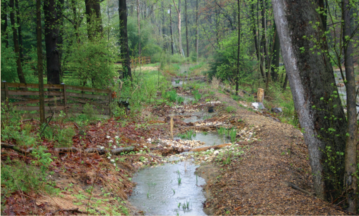
A seepage reservoir at Wilelinor Stream. The main stream channel is to the right.
