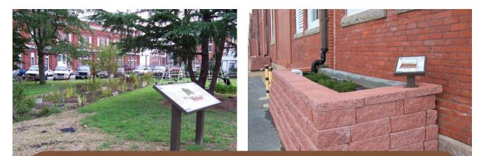
NORFOLK NAVY SHIPYARD LEFT: A bioretention facility, that was formerly an abandoned railroad line, built for treating street runoff. RIGHT: Stormwater planters treat rooftop runoff from a public works vehicle maintenance building.
